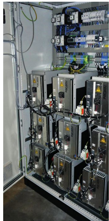
Below: “Storage battery:Former technology vs. New technology with Pacadu”. In contrast to other storage units, one single broken cell does not affect the entire network any longer with Pacadu. - Copyright: ASD Automatic Storage Device GmbH Right: A Pacadu – control box: the control electronics on top and battery cells below. – Copyright: ASD Automatic Storage Device GmbH
